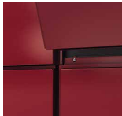
Subsequent cassette laps over neighbour at side and engages with cassette in course below.
